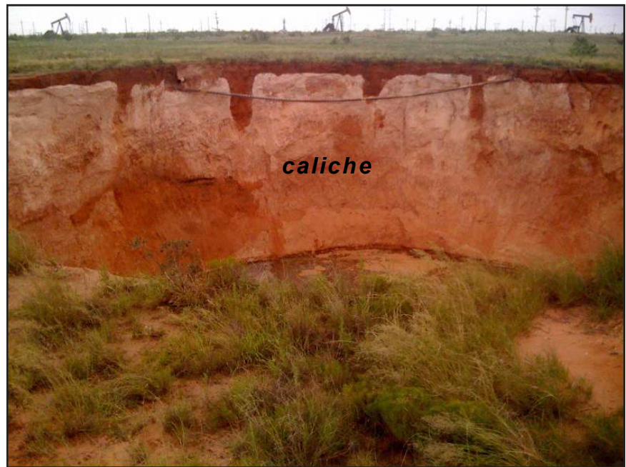
Figure 4 - Newly-formed sinkhole within an oil field near Denver City, Texas.
